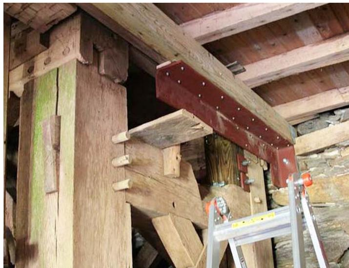
**An example of the structural work being done on some of the Grist Mill framing. The roof also needs work.**
