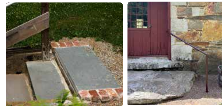
The Gurleyville Gristmill received some updates this spring! Pictured above is the new hand railing at the mill's entrance, installed by volunteer Tom DeJohn, and the new stone staircase installed by Peter Baldwin. Thank you to Tom & Peter for their time and craftsmanship!
