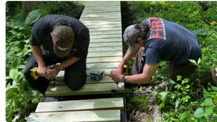
Stewardship staff replaced the boardwalk at Knowlton Hill Preserve in Mansfield earlier this spring.
